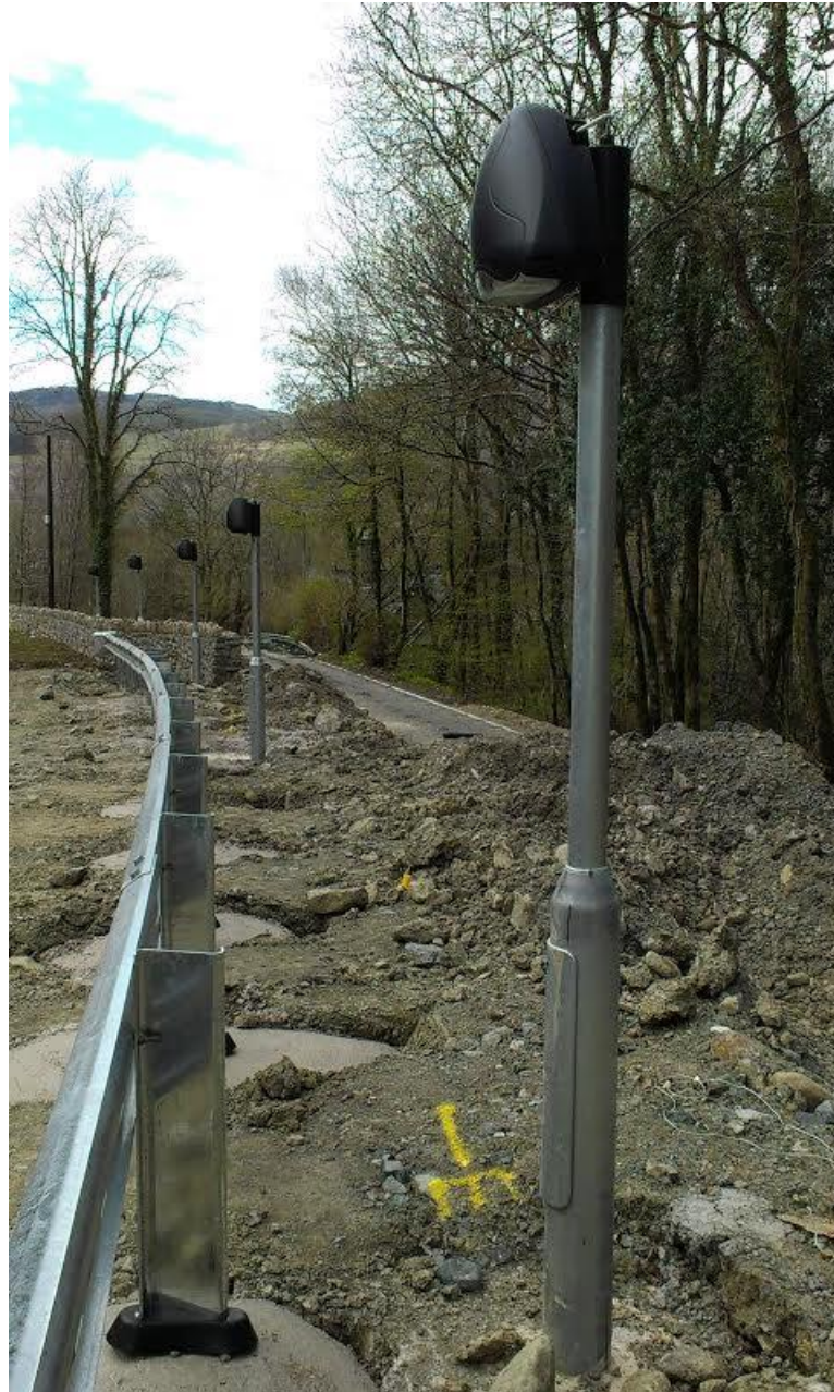
Figure 6.6. Down lights installed to reduce spill on A470 Cross Foxes to Maes-y-helmau, Wales (©Jill Jackson)
