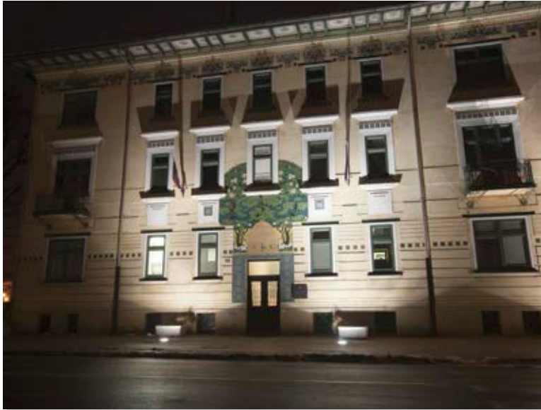
Lamps mounted right against the façade cause shadows which do not give the feeling of authenticity of the object.
