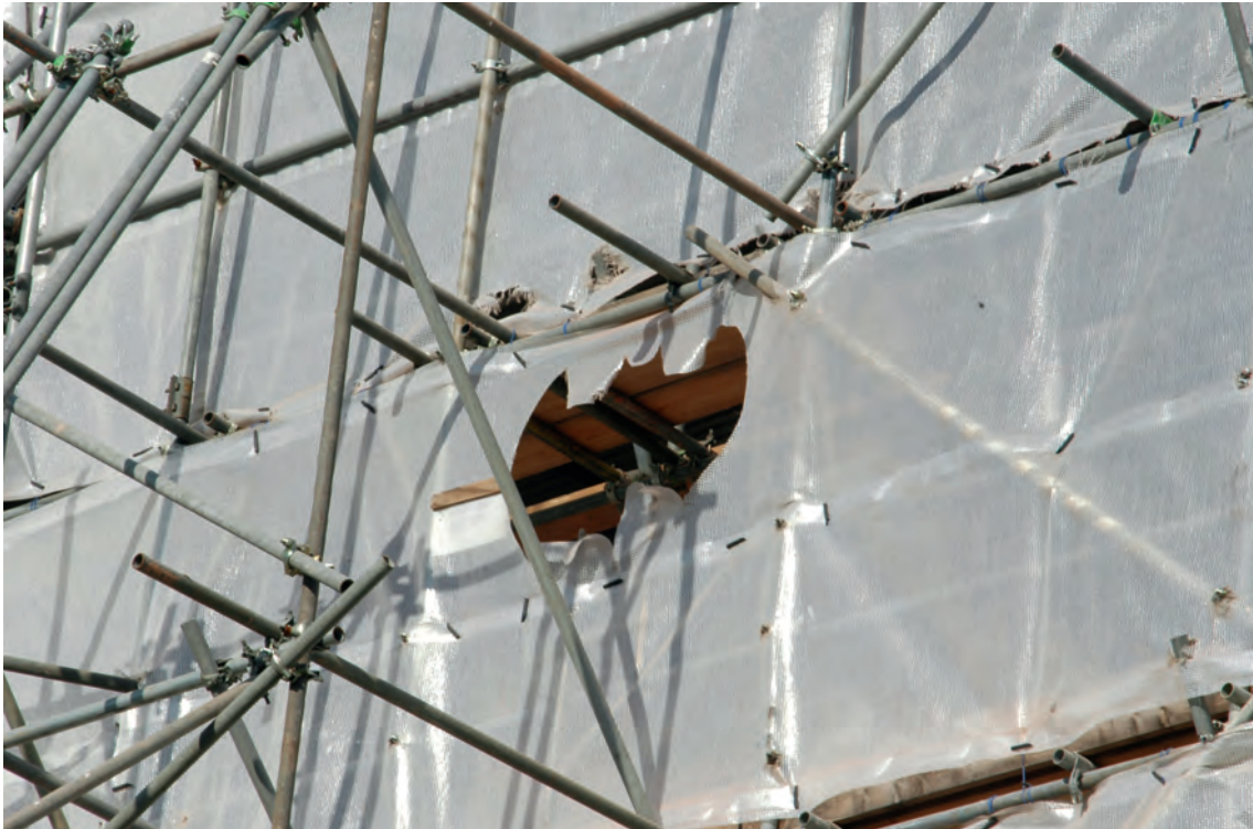
Position scaffolding around a bat route/exit and create gaps for them. (© Phil Richardson)
