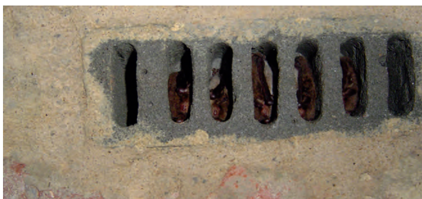
Bat brick in situ in tunnel roof. (Keith Zealand)
